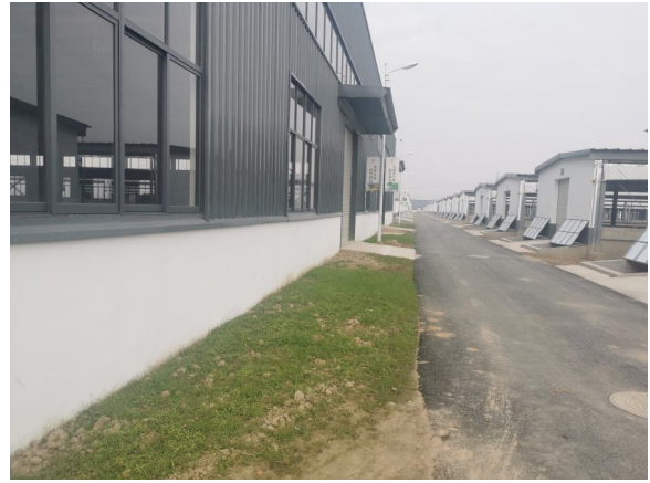
饲料工车间现状
